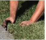
TIP: DO NOT BACKFILL WITH SOIL WITH HIGH CLAY **CONTENT.** Water must be able to easily pass through the backfilled soil.
