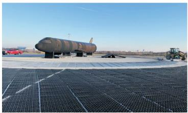
In addition, the pavers could handle temperatures upwards of 325°F before any type of damage or deformity occurs, an optimal solution for firefighting scenarios.
