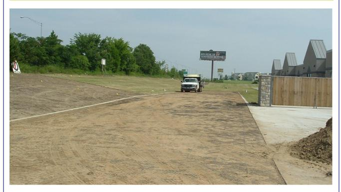
During the installation: Tufftrack Grassroad Paver panels were connected, filled, and leveled in the designated fire lane areas.
