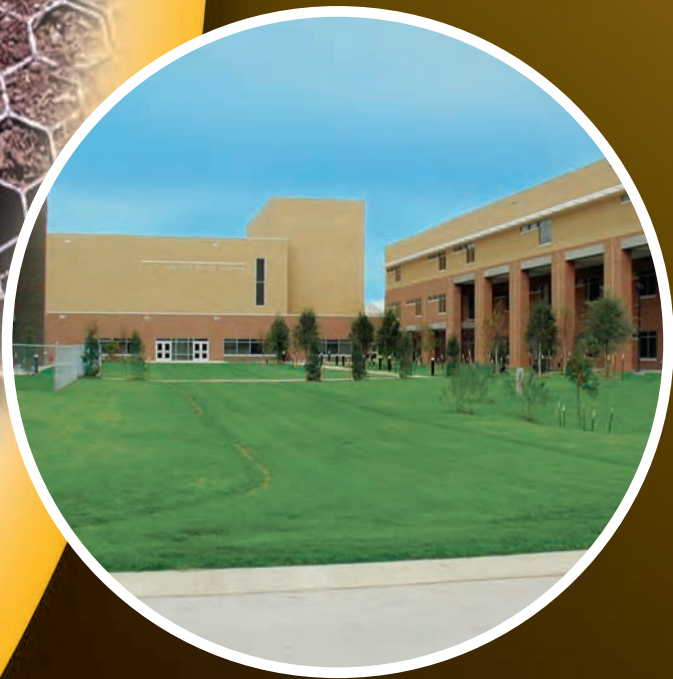
Brewer High School before and after Tufftrack™ Installation
