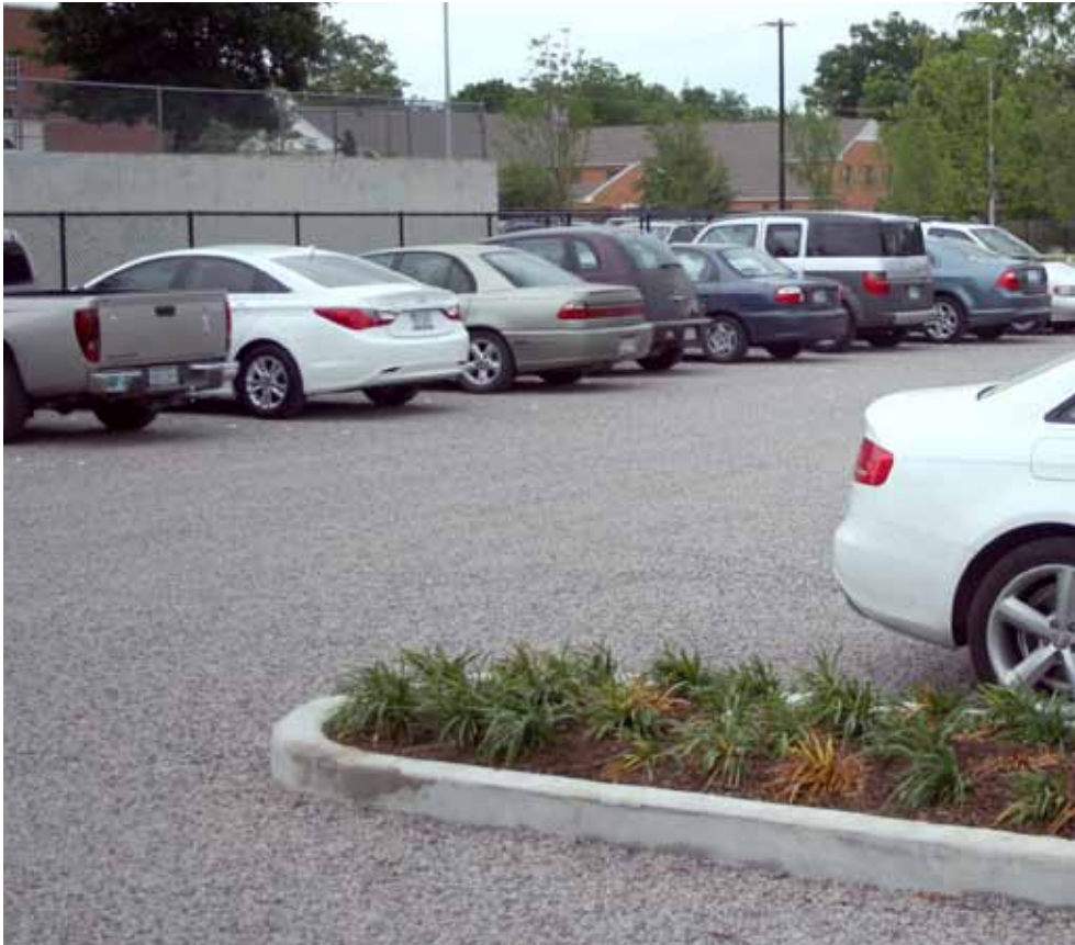
EZ Roll™ Gravel Paver with geotextile fabric backing.
