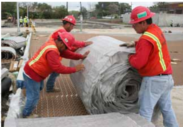
Above Photos: Installation of NDS EZ Roll Gravel Paver and EZ Marker Parking Delinators.
