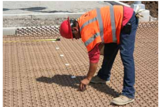
Above Photos: Installation of NDS EZ Roll Gravel Paver and EZ Marker Parking Delinators.
